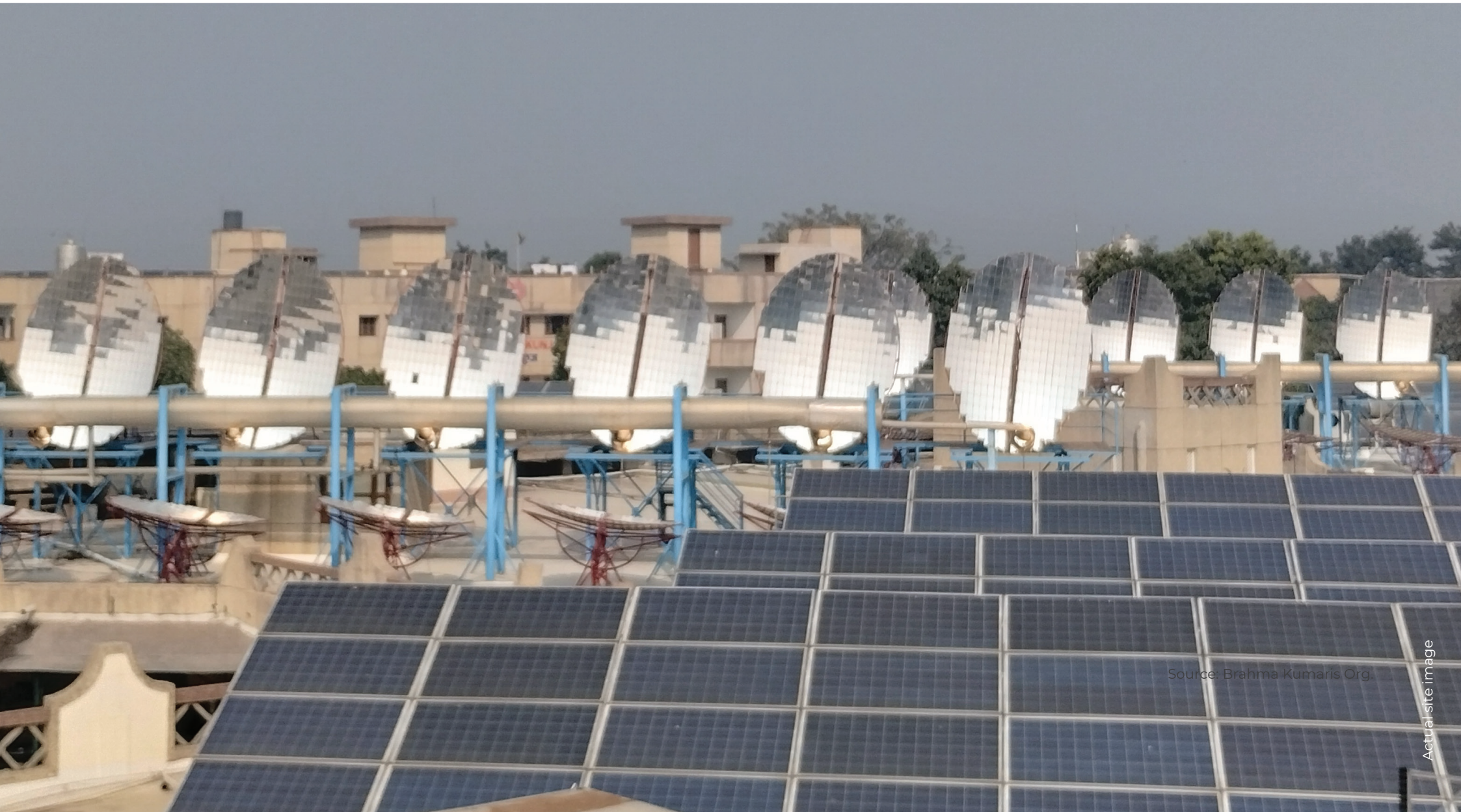
Figure 2: Solar panels installed on Om Shanti Retreat Centre rooftops (concentrated solar thermal project in the back)
